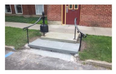
The bluestone stairs on the Chestnut Street side have been repaired – the bottom stone was replaced and the top stone reset. Because they were angled incorrectly, last year water lay in the one closest to the street and would freeze causing obvious problems. Cooper VanCott, who put in our bell tower blue stone stairs, is a bluestone craftsman.
